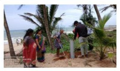
Explanation: The pipes are buried securely with 6-12 inches remaining above ground, ensuring stability.
