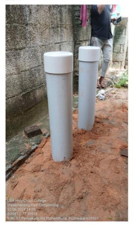
Explanation: Holes are drilled at intervals of 6 inches to ensure proper aeration within the composting pipe.
